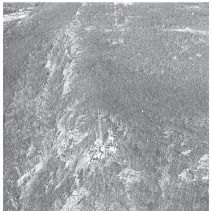
Fig. 5. Broadcast and microwave towers dominate the skyline of a community.
